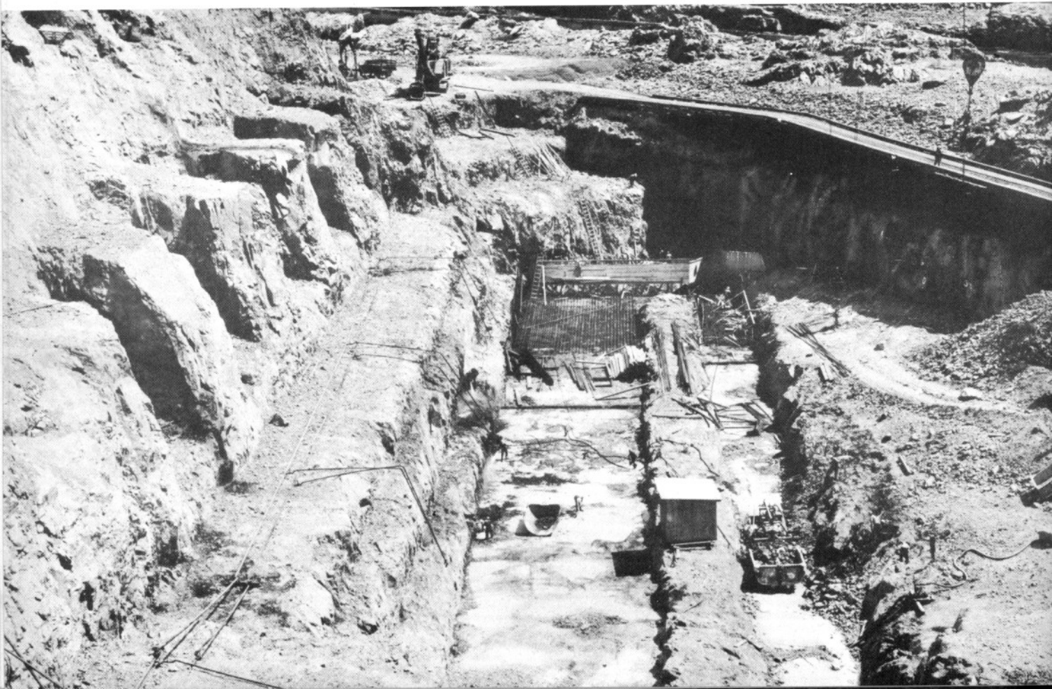
Excavation for the Powerhouse
