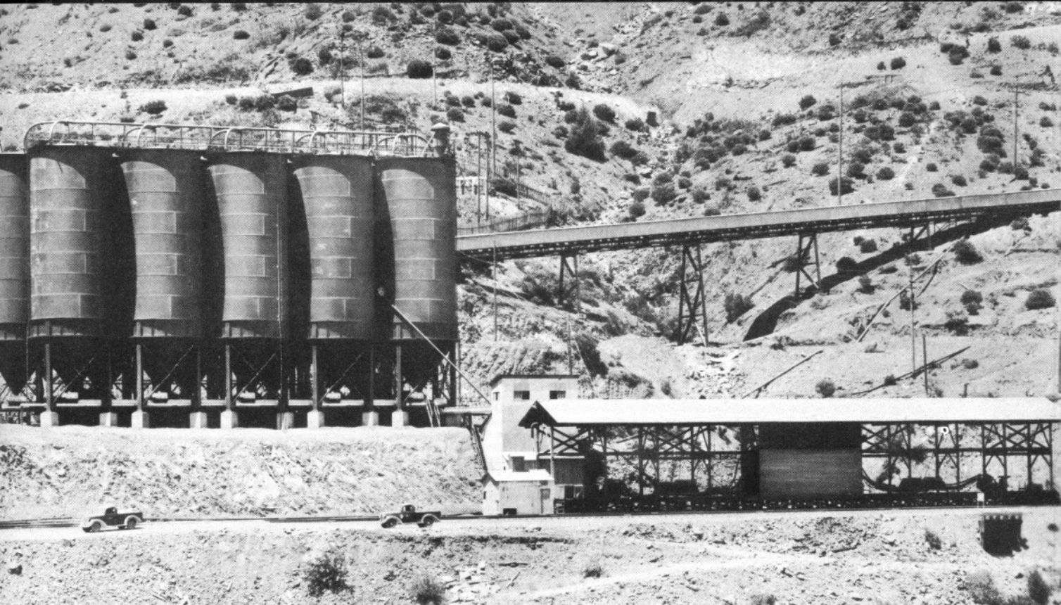
Cement unloading and storage facilities
