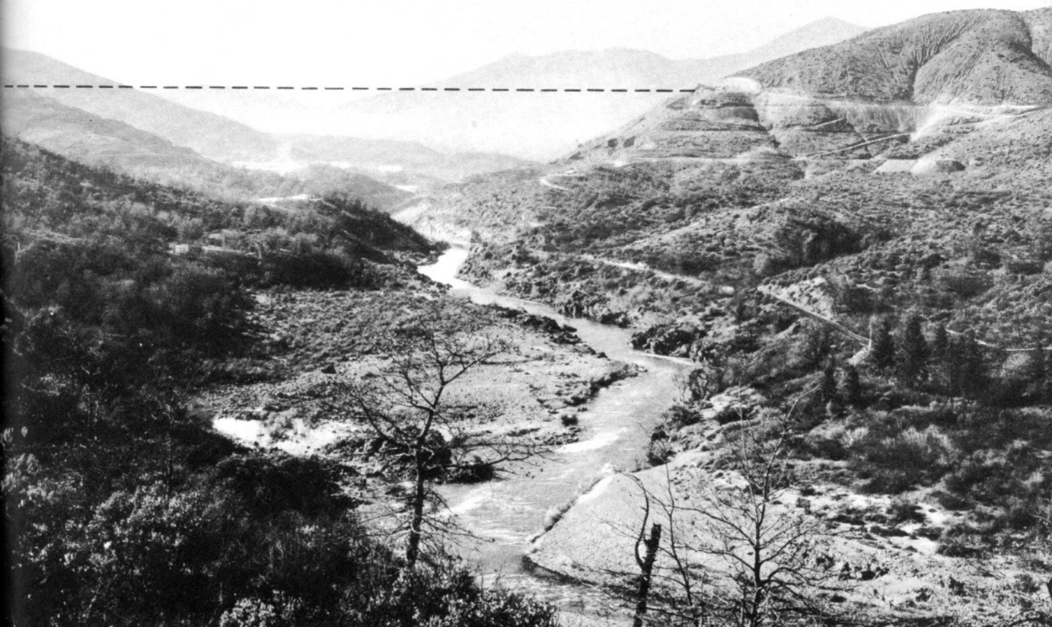
Damsite looking downstream January, 1939
