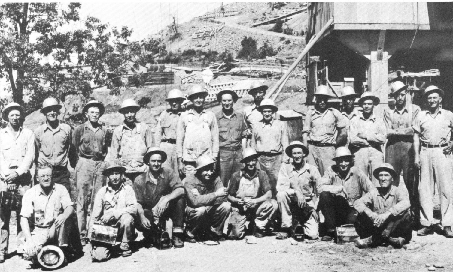
Powerhouse Carpenters: Chas. Silva, Foreman (seventh from left, standing)
