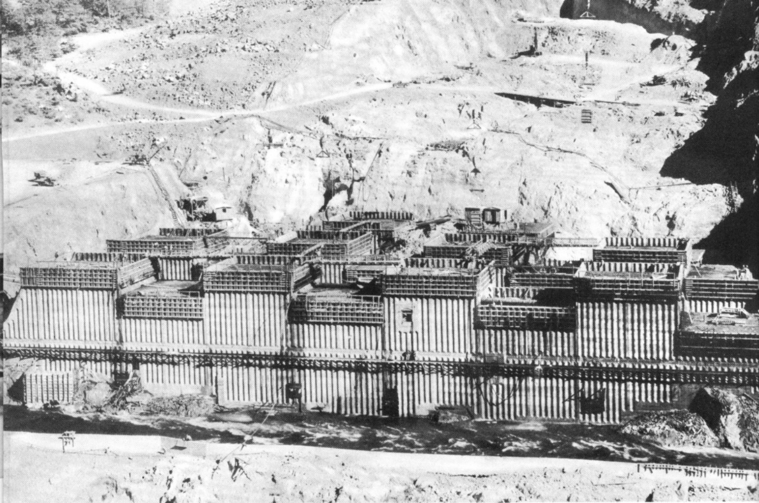
Early stage of concrete work, East Abutment—September, 1940
