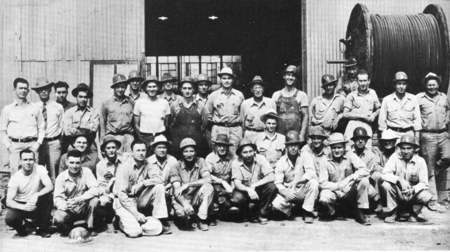
Electrical Department: L. E. Osborn, Chief Electrician (fourth from right, kneeling, front row)
