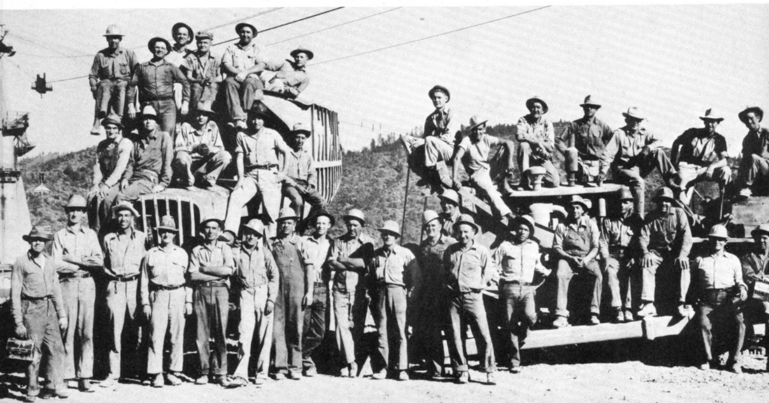
Excavation Crew: J. P. Riley, Foreman (second from left, front row); Dale Bryant, Foreman (third from left, front row); A. M. Brown, Foreman (fourth from left, front row); Jess Withers, Foreman (sixth from left front row)
