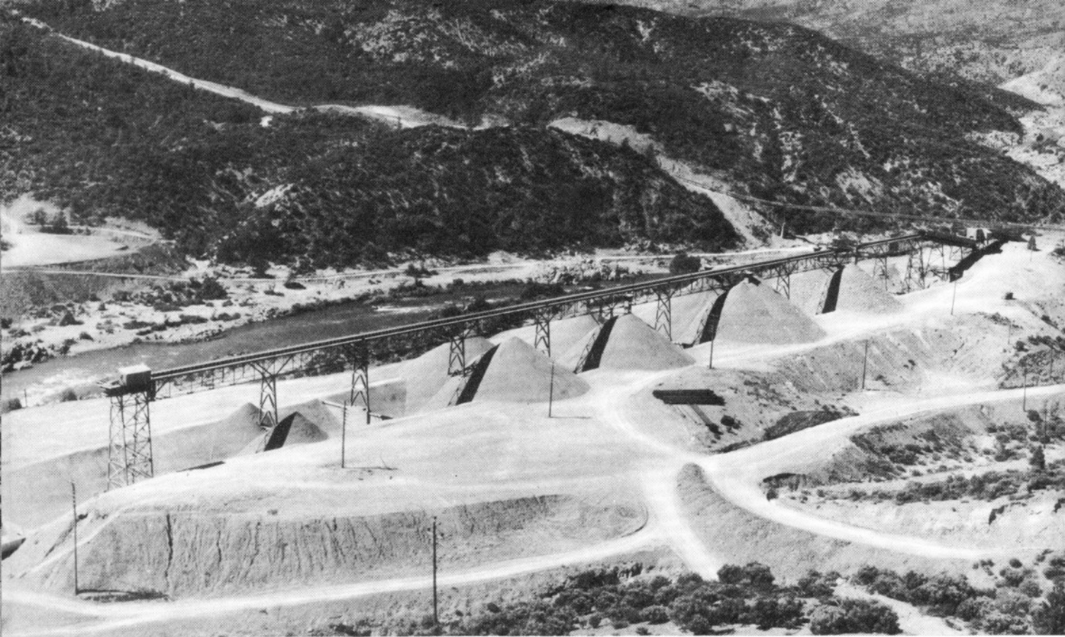
The aggregate stock pile
