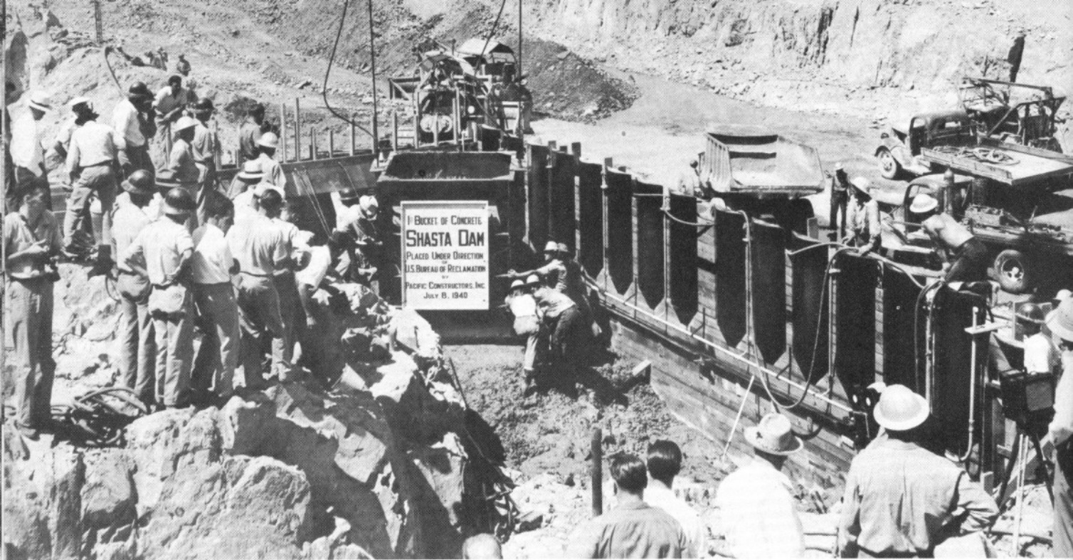
Placing the first bucket of concrete
