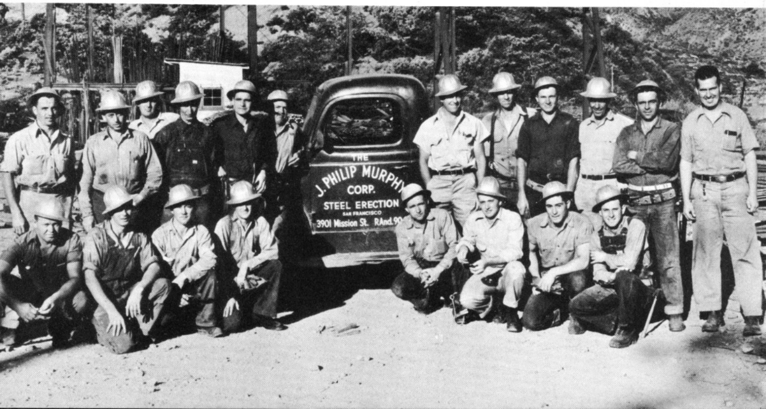
Reinforcing Steel Crew (The J. Philip Murphy Corp., Sub-contractors): Don Rutherford, Superintendent (sixth from right, standing); Frank Skoubege, Assistant Superintendent (first at right, standing)
