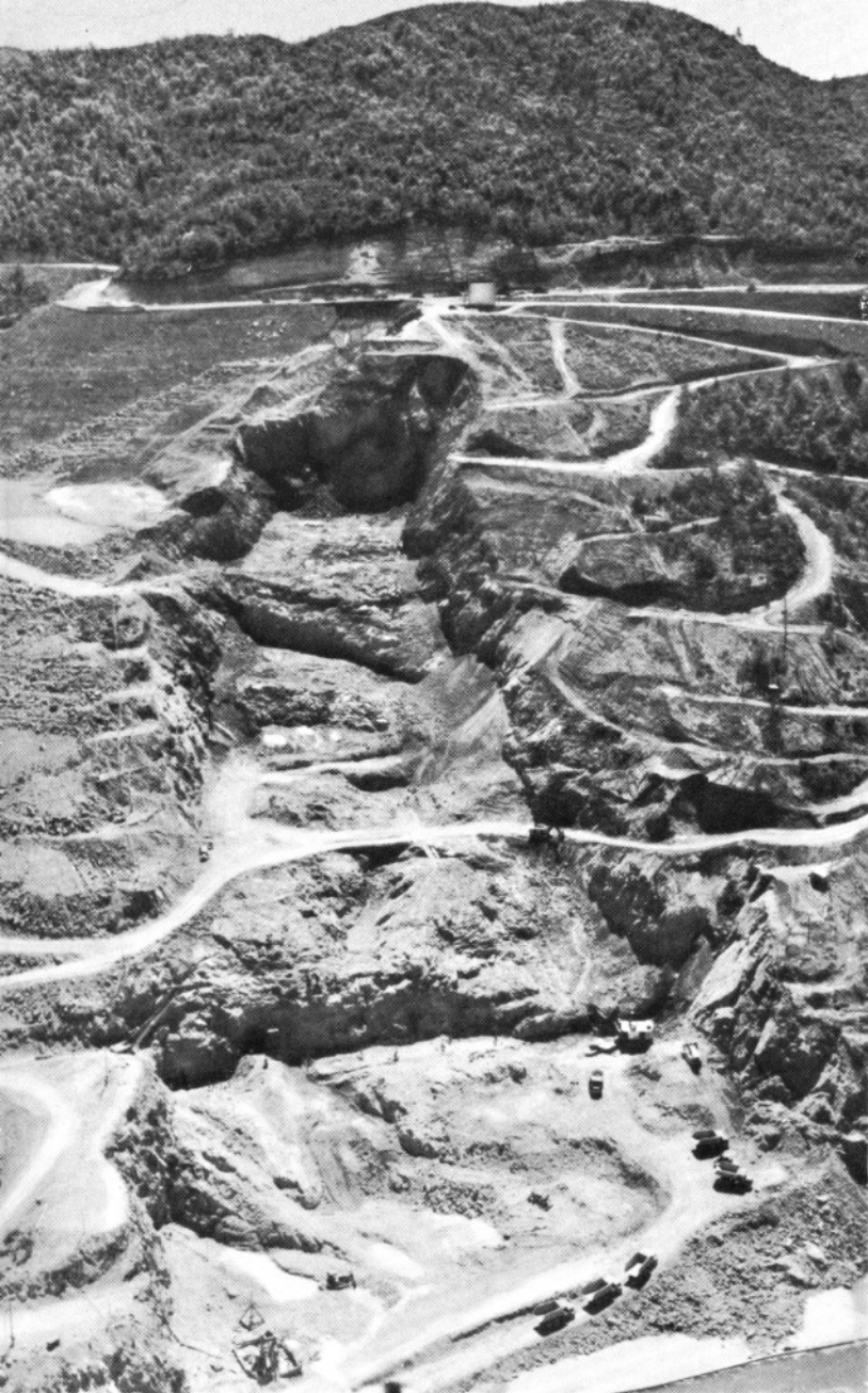
East Abutment key way excavation near completion
