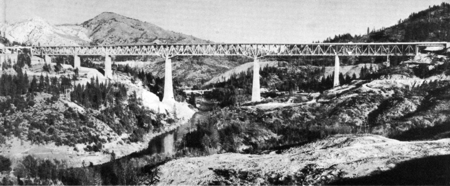
The Pit River Bridge
