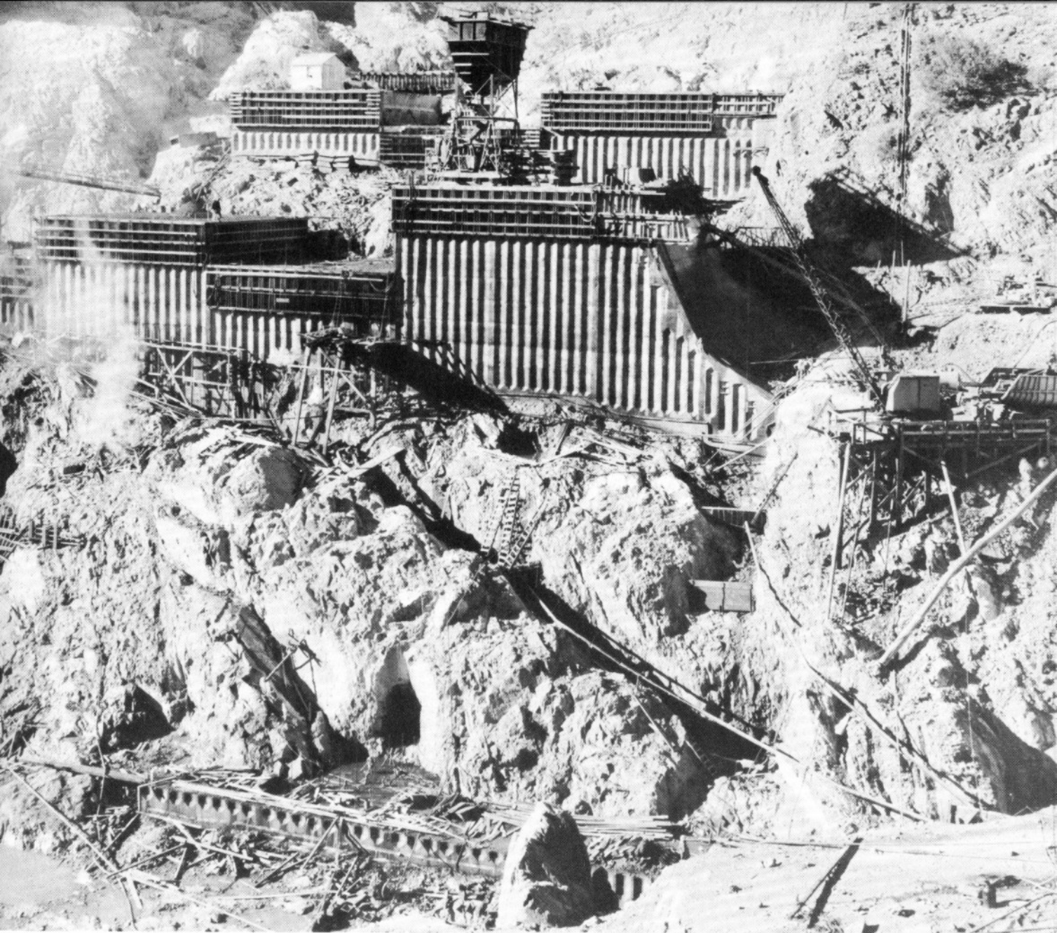
Note soft seams which had to be dug out
