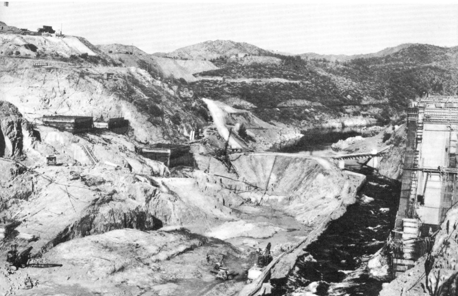
Pumping out and excavating "The Hole"—Note fill Cofferdam for diversion—November, 1940
