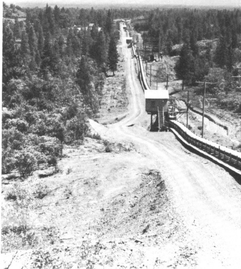
Section of world's longest conveyor belt system—Redding to Shasta Dam
