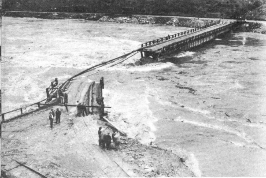
Main truck bridge at peak of 1940 flood
