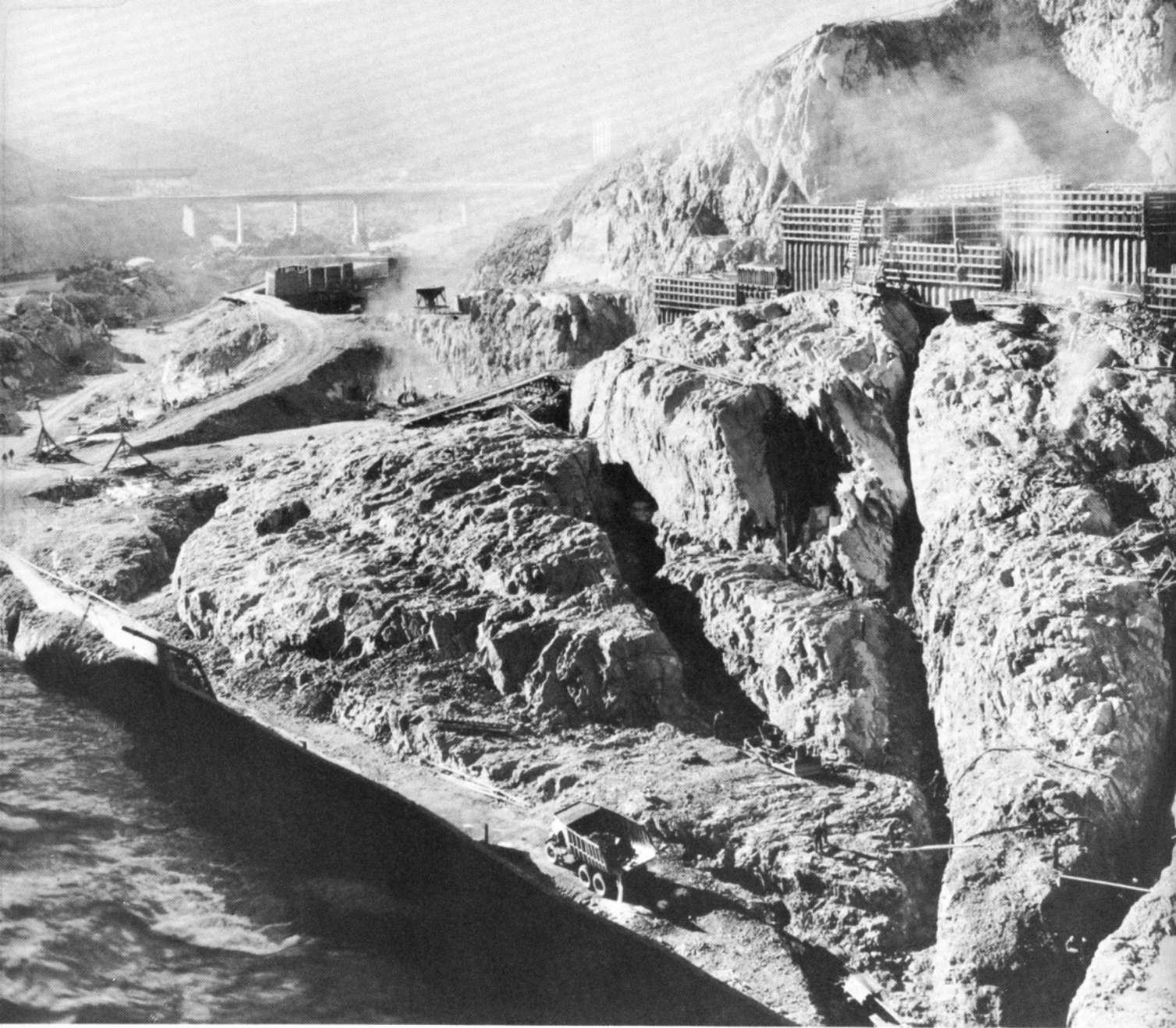
Excavation near bed of river—
