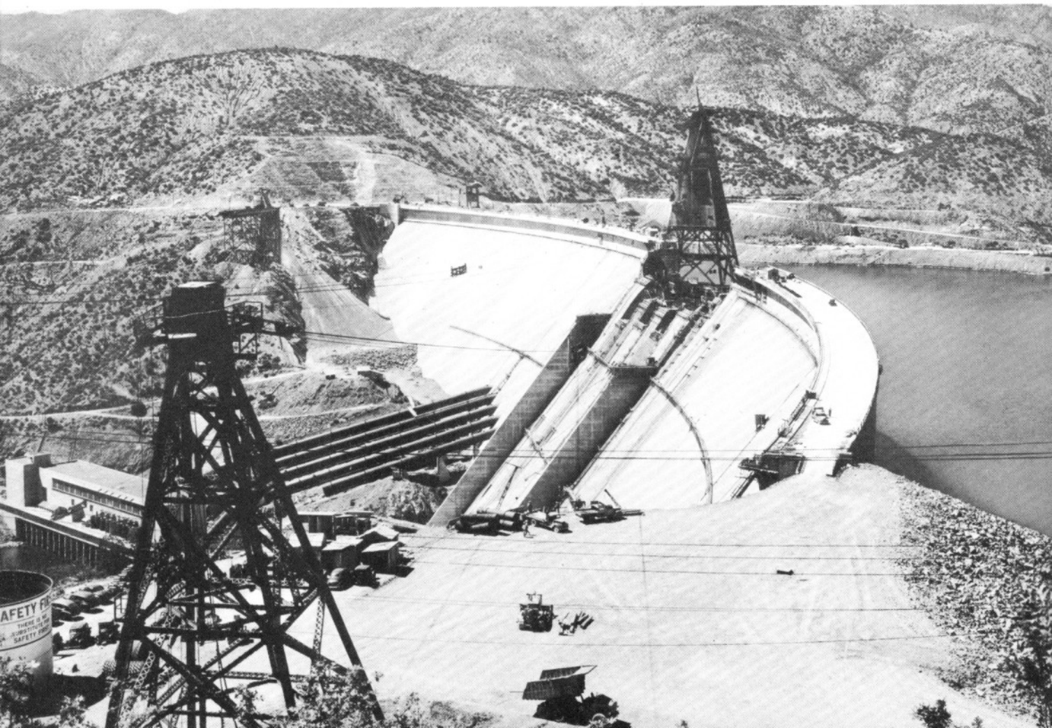
View from left abutment as dam nears completion—September, 1944
