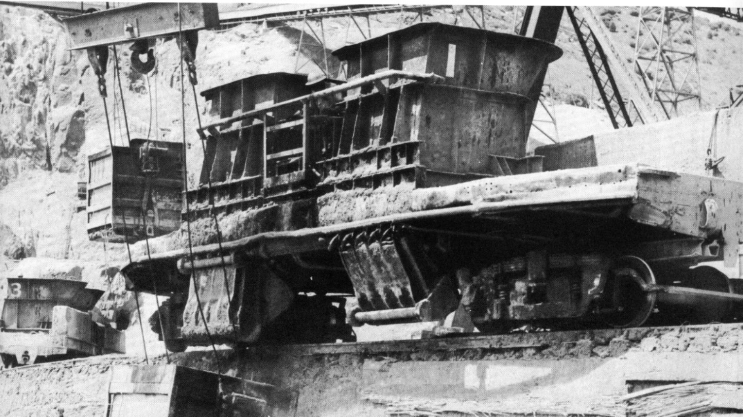
The "Goose Car" loading an 8-yd. bucket
