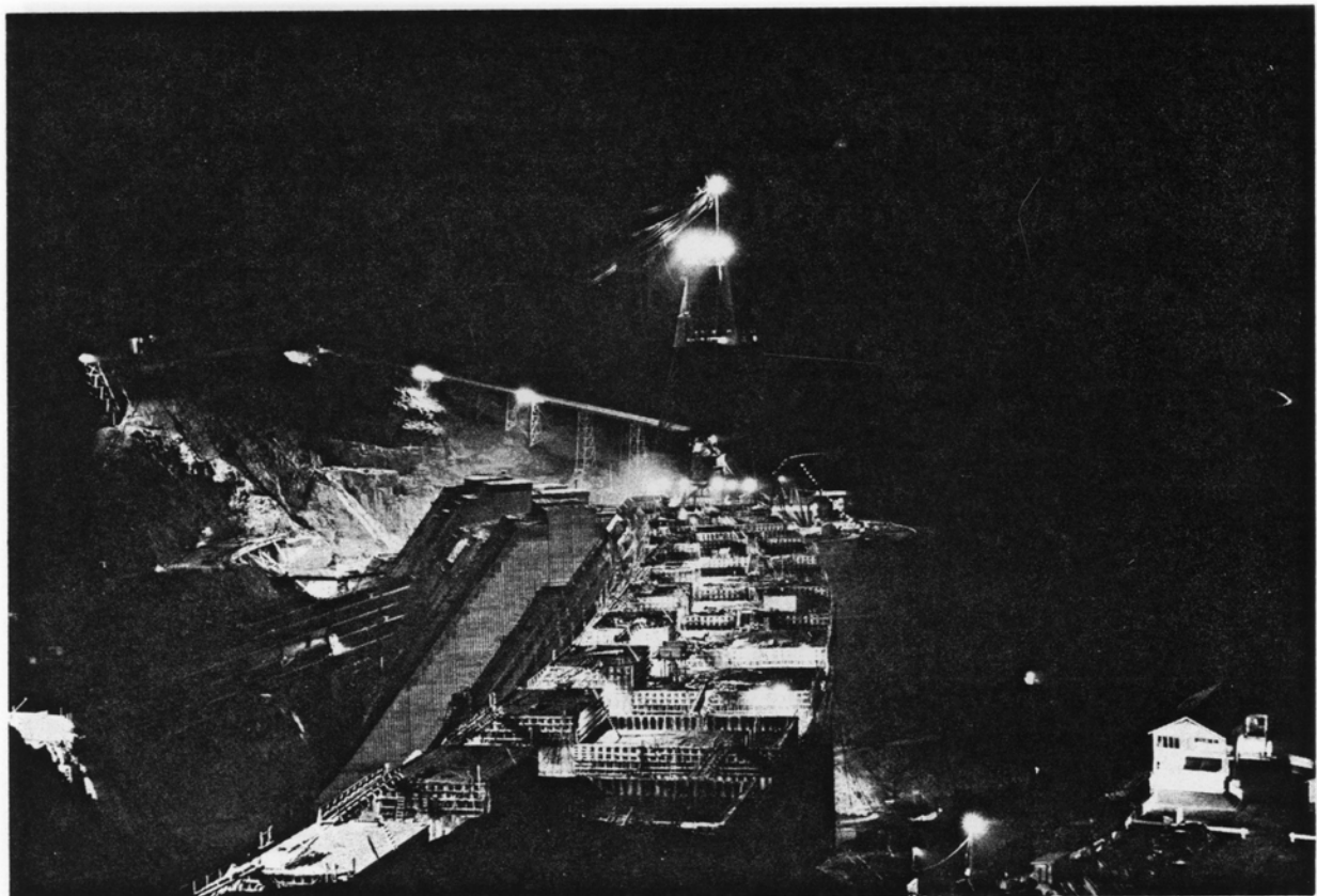
Work is carried on around the clock to rush completion of the Bureau's monumental Shasta Dam containing 6,535,000 cubic yards of concrete.
