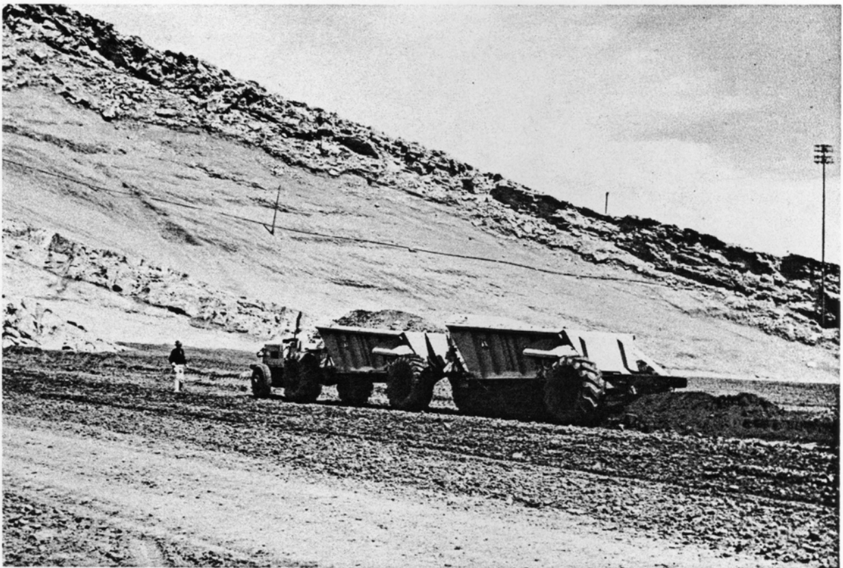
Tandem Euclids dump 40 tons of earth rock for Horse Tooth Dam.
